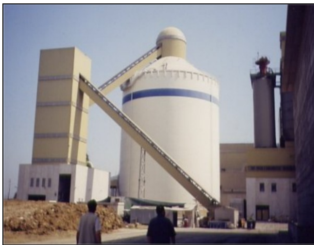
Figure 3.2.74. Silo de clinker.
