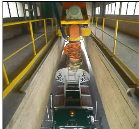
Figure 3.2.80. System for the bulk loading of cement.
