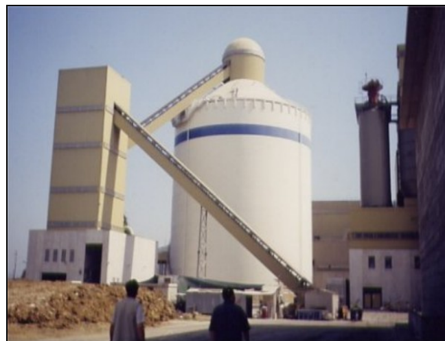
Figure 3.2.74 Clinker storage silo.
